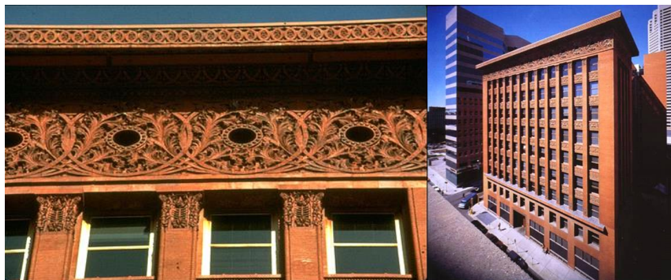
Figura 55 - Wainwright Building – Louis Sullivan
